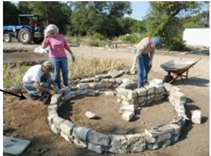
Sherry critiques the masonry work –
